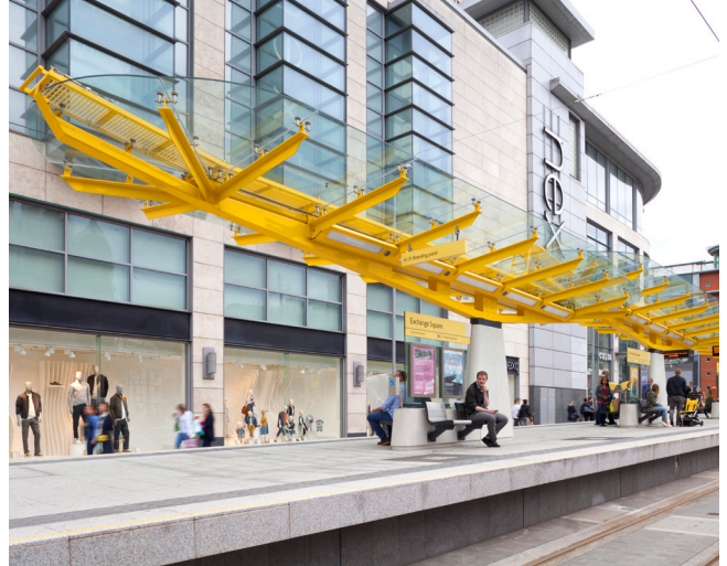
Exchange Square: Dellner Glass Solutions supplied toughened, laminated, shaped glass canopies for the tram stations at Manchester's Exchange Square.
